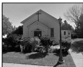
St. Andrews Church Sackets Harbor
